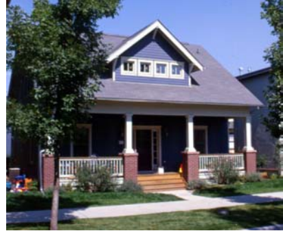
This new bungalow home in is similar in style and scale to many existing bungalow homes in Pottstown's Rosedale section.
