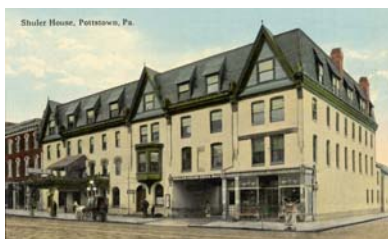
Left, the Shuler House was demolished for urban renewal; the house at right was demolished for a pizzeria.
