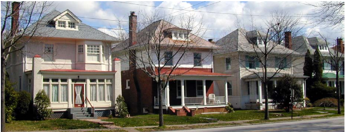
These early 20 th century homes along High Street are similar in height and mass and are spaced evenly, giving the block a pleasing appearance.
