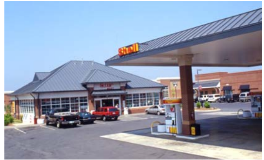
This convenience store, with an island for dispensing gasoline, is built of brick, with a standing seam hip roof, making it compatible with traditional neighborhoods.
