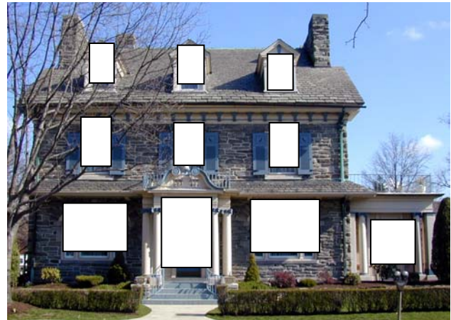
This building has a wall to opening ratio of 1 to 1.
