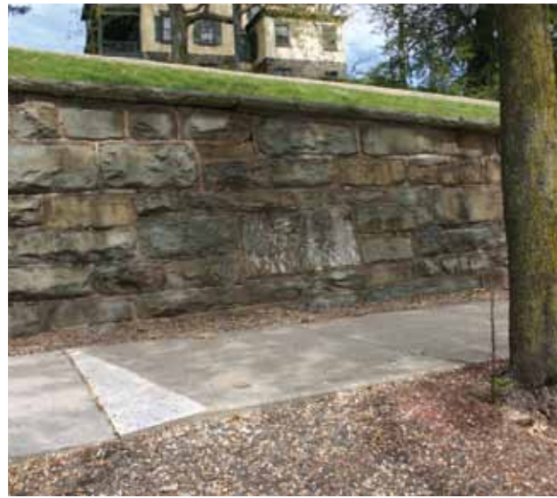
This is a completed sidewalk repair in front of the Hill School in Pottstown.
