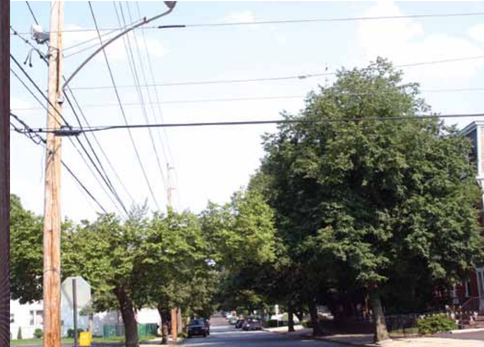
If a tree potentially grows high enough to reach its wires, PECO trims tree branches a set distance away from their wires, depending on the species of tree and the voltage running through the wires. Above, the linden trees on the left have been given a "flat top" cut more than 15 feet below the closest energized lines. Note the contrast with the appearance of the uncut linden trees on the right side of the street.
