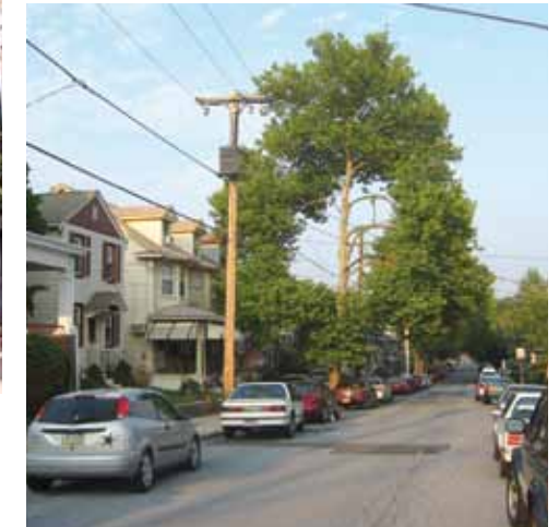
If a tree potentially grows high enough to reach its wires, PECO trims tree branches a set distance away from their wires, depending on the species of tree and the voltage running through the wires. Above, the linden trees on the left have been given a "flat top" cut more than 15 feet below the closest energized lines. Note the contrast with the appearance of the uncut linden trees on the right side of the street.
