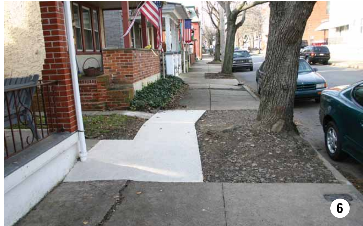
1. A badly heaved sidewalk in Pottstown was repaired by enlarging the tree well and replacing the concrete sidewalk with asphalt.
