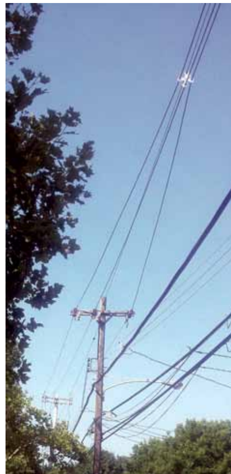
BELOW RIGHT - Thanks to bundled wiring, this maple tree is growing up and around the electric line. If there were a number of these trees in a row, the utility line would be almost invisible from the street.
