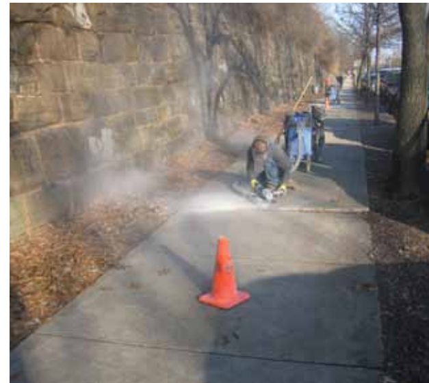
Using special saws, sidewalks can be repaired in a few minutes. More than 50 sidewalks can be repaired in a day. It is favored by agencies like housing authorities and colleges because it is far less expensive and messy than removing and replacing concrete.
