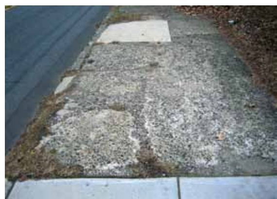
Concrete sidewalks are also susceptible to spawling.
