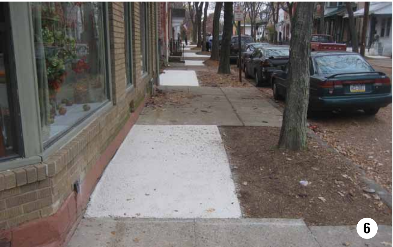
1. Asphalt was used to replace 11 broken concrete sidewalks in another Pottstown demonstration project.
