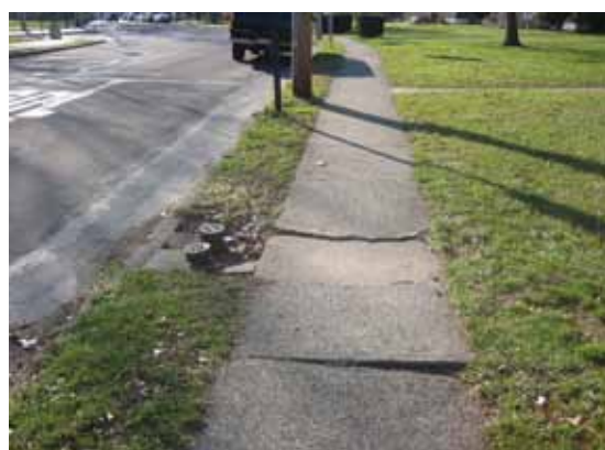
Tree roots are only one cause of lifted sidewalks. Most sidewalks are lifted because of freezing and thawing ground or the improper installation of underground pipes.
