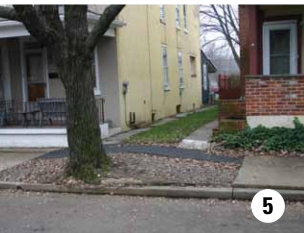
1. A badly heaved sidewalk in Pottstown was repaired by enlarging the tree well and replacing the concrete sidewalk with asphalt.
