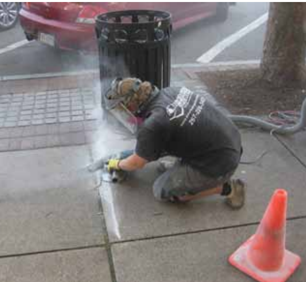
Rather than remove lifted concrete panels, lifts of 2 inches or less can be beveled by a firm called Always Safe Sidewalks. Using a patented technology, the firm can remove the trip hazard and keep the sidewalk compliant with ADA standards.
